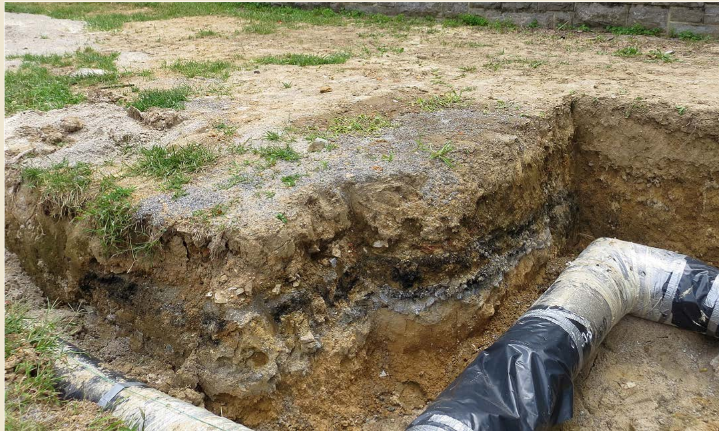
This site is a good candidate for SPR because soil is compacted and has an impermeable layer that can likely be broken up by the backhoe subsoiling process. Note limestone gravel mixed in soil indicates pH will be high, which will not be altered by the rehabilitation process. Surface gravel should be removed if possible and underground infrastructure clearly marked. Photo by Susan D. Day
