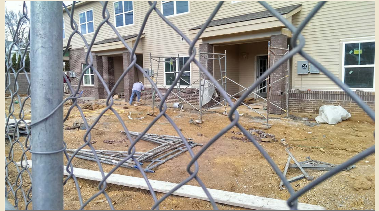
After construction this area will be planted with trees, shrubs, and turf. Heavy grading and a confined building site have resulted in severe soil compaction that is a prime candidate for SPR. Photo by Susan D. Day
