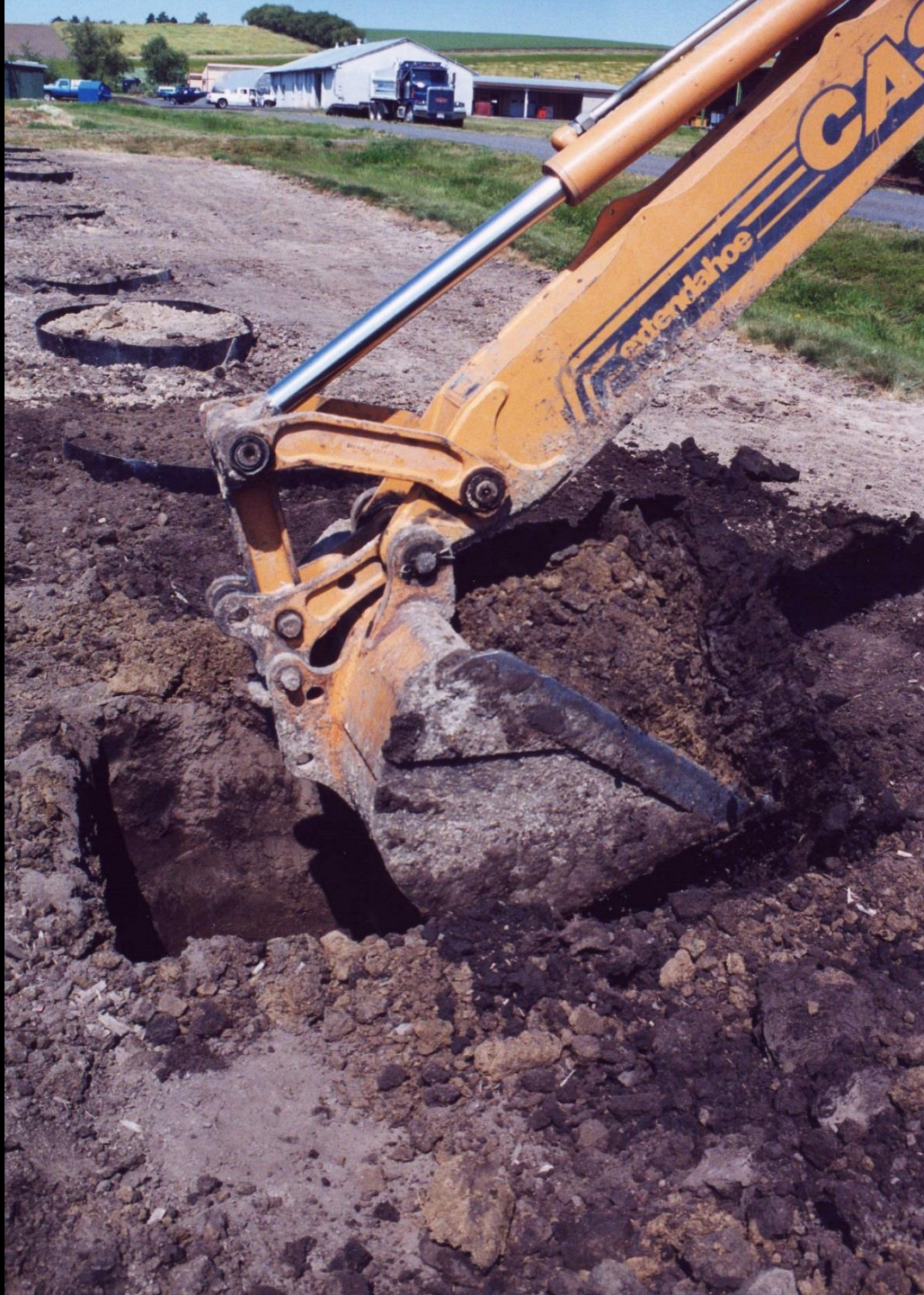
Sub-soiling with a backhoe at U. Idaho experimental farm near Moscow, ID (Scharenbroch)
