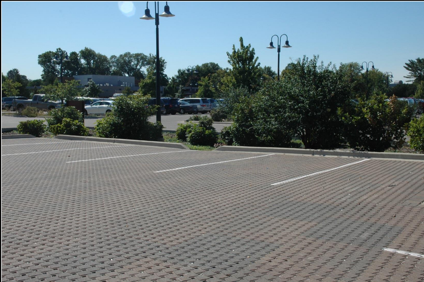
Permeable paver and bioswale parking lot at The Morton Arboretum in Lisle, IL
