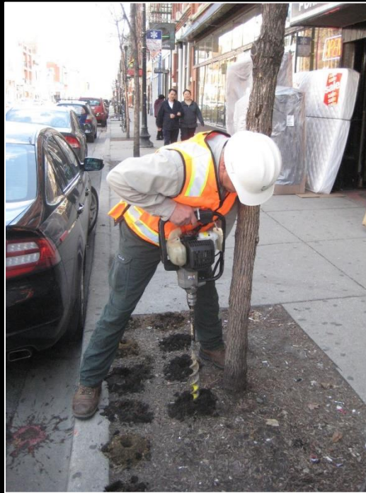
Radial trenching, drilling, and high-pressure air tillage
